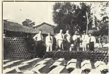
Fig. 3. Concrete inverts and pipe made in the "Plantel" at San Miguel, Republic of El Salvador. The pipe was used for subsoil drainage.
